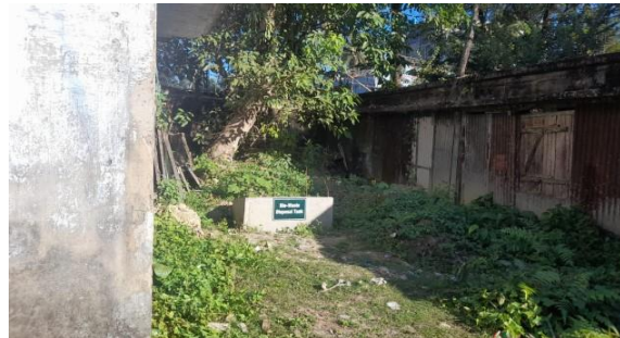
Bio-Waste Disposal Tank
