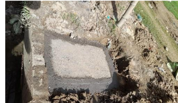
Ground Water Recharge Pit
