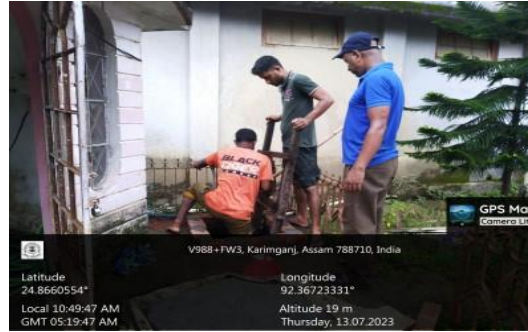
Cleaning of reservoir and overhead tanks
