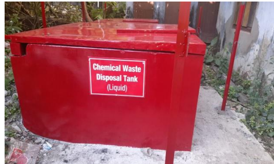
Chemical Waste Disposal Tank(Liquid)
